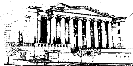
ALABAMA JUDICIAL BUILDING
